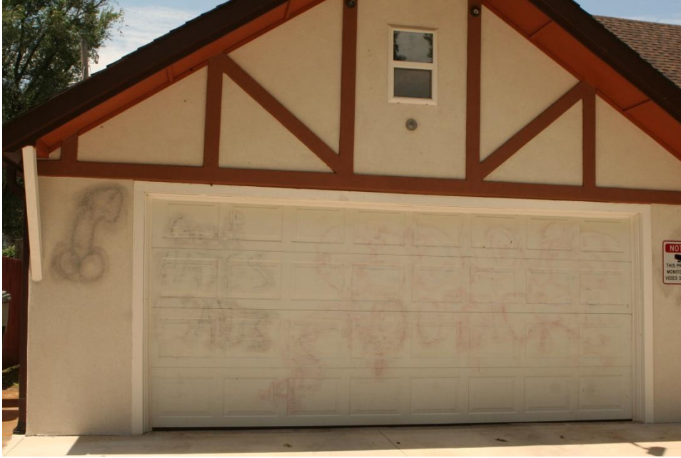
Figure 60. Westboro Baptist Church property was vandalized in May 2010. Church members initially left the graffiti, which included sexually explicit images and misogynistic language, to illustrate, they said, the depravity of the Topeka community. By mid-summer, though, they had painted over the images, though they were still largely visible. July 18, 2010 photograph courtesy of Ailecia Ruscin. All rights reserved.
