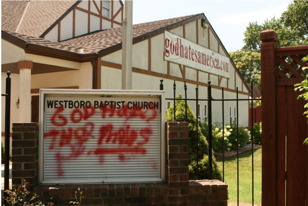
Figure 2. Westboro Baptist Church is attached to the modest home of Fred Phelps, Sr. and his wife Margie. The front of the building is covered with a massive banner promoting the church's flagship website. A privacy fence runs the perimeter of the block, which includes homes owned by church members. The church's sign was long ago vandalized with graffiti that proclaims "God Hates the Phelps." Photograph courtesy of Ailecia Ruscin, July 18, 2010. All rights reserved.
